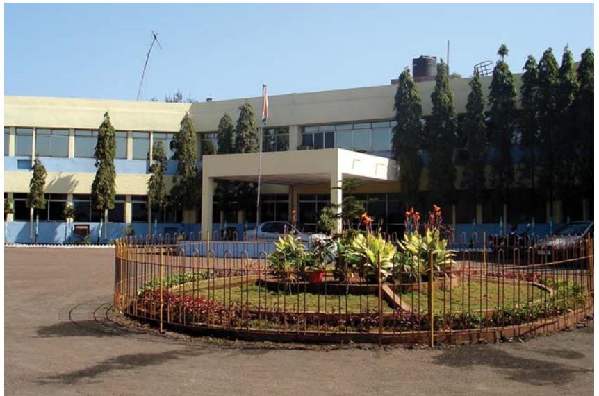
Tata Metaliks' pig iron facility at Redi, Maharashtra
