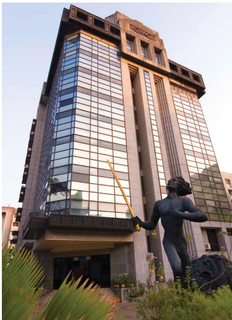
CMC's Mumbai office is designed for increasing energy efficiencies
